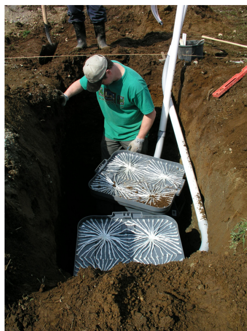
Figure 2. 64 samplers were installed under raspberry rows and alleys to catch water leaving the root zone. Photo by Shawn Kuchta.
