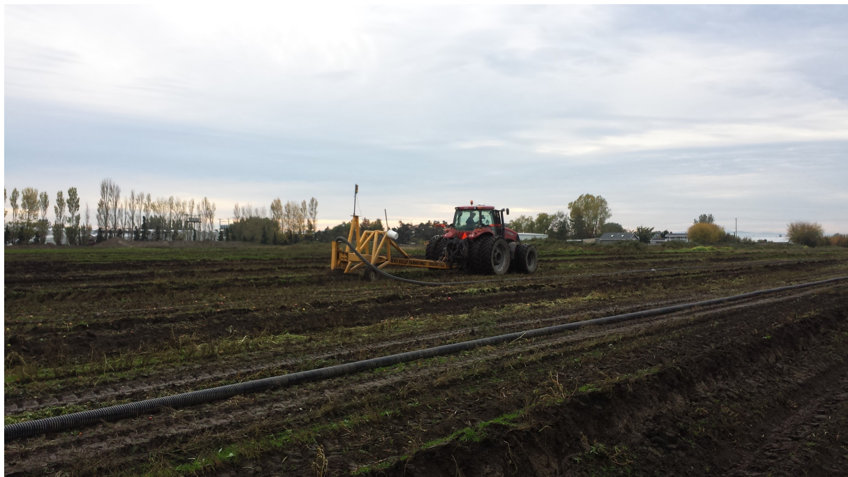
Figure 3 Tile drainage installation by collaborating farmer at the field-scale demonstration and research site
